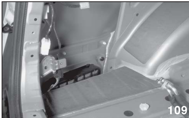
Rear Evaporator Removed
